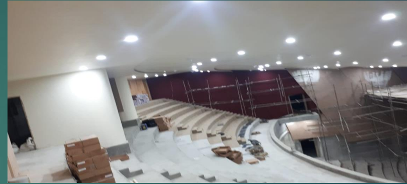
17. Up Lifting of Sir Syed Auditorium , Mangla Cantt
